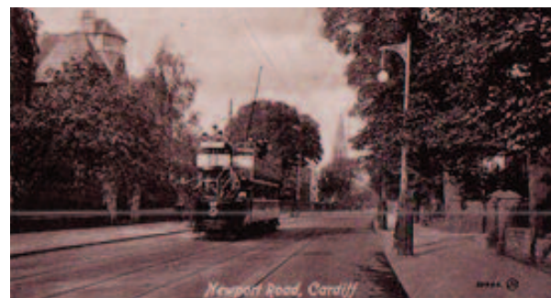
Figure 1. A tram running along Newport Road in Cardiff 2
